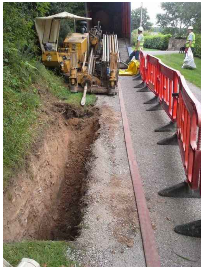
Drilling Rig/Launch Pit
